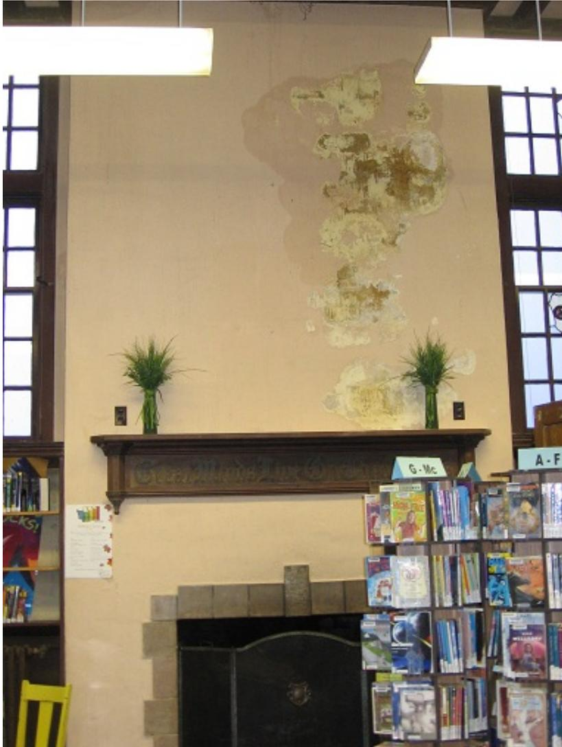
Plaster throughout the main public areas on both floors as well as the entrance, foyer, bathrooms, conference room and children's room will be repaired and where necessary replaced. The project will include demolishing delaminated plaster, re-lathing, reframing and re-plastering. Cracks and seams will be filled and new paint applied. Shane Moncy of Coastline Roofing Systems of South Bend will perform the work.
